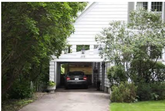
A property demonstrating a porte cochere.
