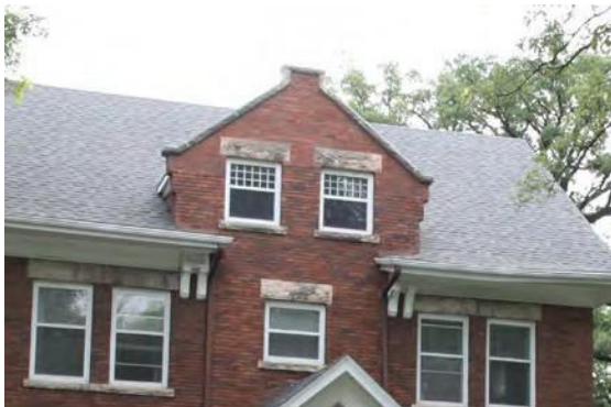
A distinctive roof form and dormer window, with prominent sills and a red masonry facade.
