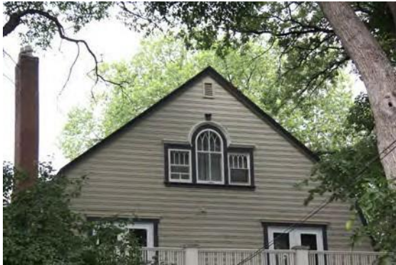
Maintain roof form and distinctive window surrounds.
